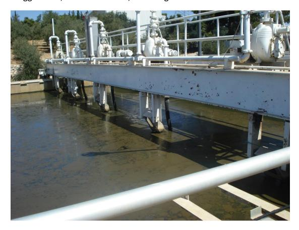
Purpose of this stage is to remove the smaller particles that wouldn't originally settle fast enough, by making them into larger particles with lower settling times.
